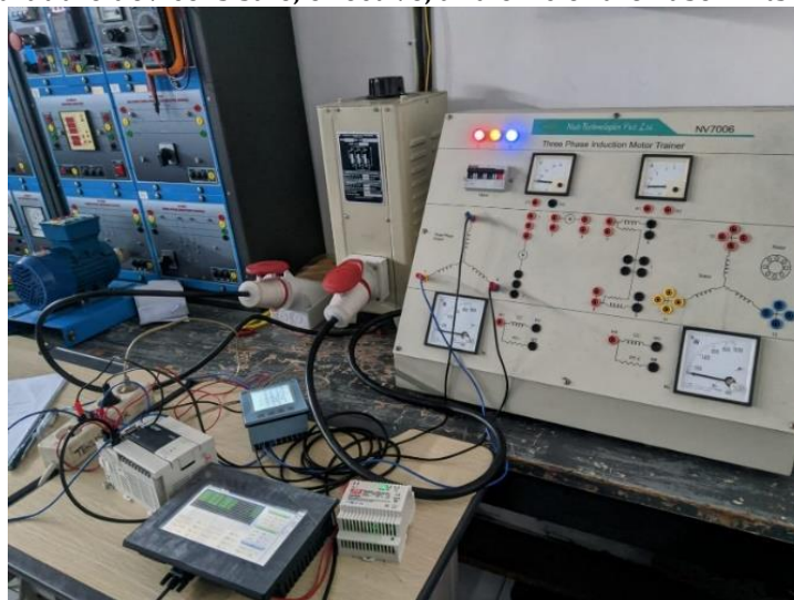
Figure 15. Testing Undervoltage, Overvoltage, Frequency
